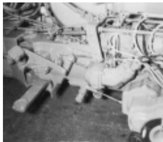
Picture 2.4: Vibrations, dirt, and temperatures up to 266°F characterize the area surrounding the engine
